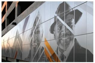
Dri-Design with Perforated Imaging uses advanced computer based manufacturing to create complex images using perforations. By varying the size, location and density of the perforations, areas of light, dark and shades in between are created to form an image. These perforations also allow the panel to provide needed airflow and/or shade to a structure. Since the images can be created from any digital picture, you are only limited by your imagination.
