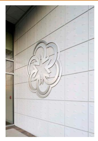
With our Embossed Panel, there is essentially no limit to the design possibilities or applications. Almost any shape or feature, convex or concave, can be embossed into the Dri-Design panels to create a distinctive, three dimensional accent.
